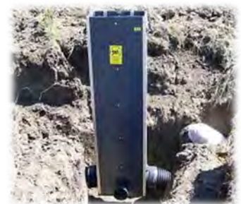
Drainage Water Control Structure
