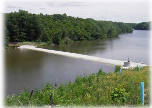
Low-flow/in-lake dam; Otter Lake, Illinois
